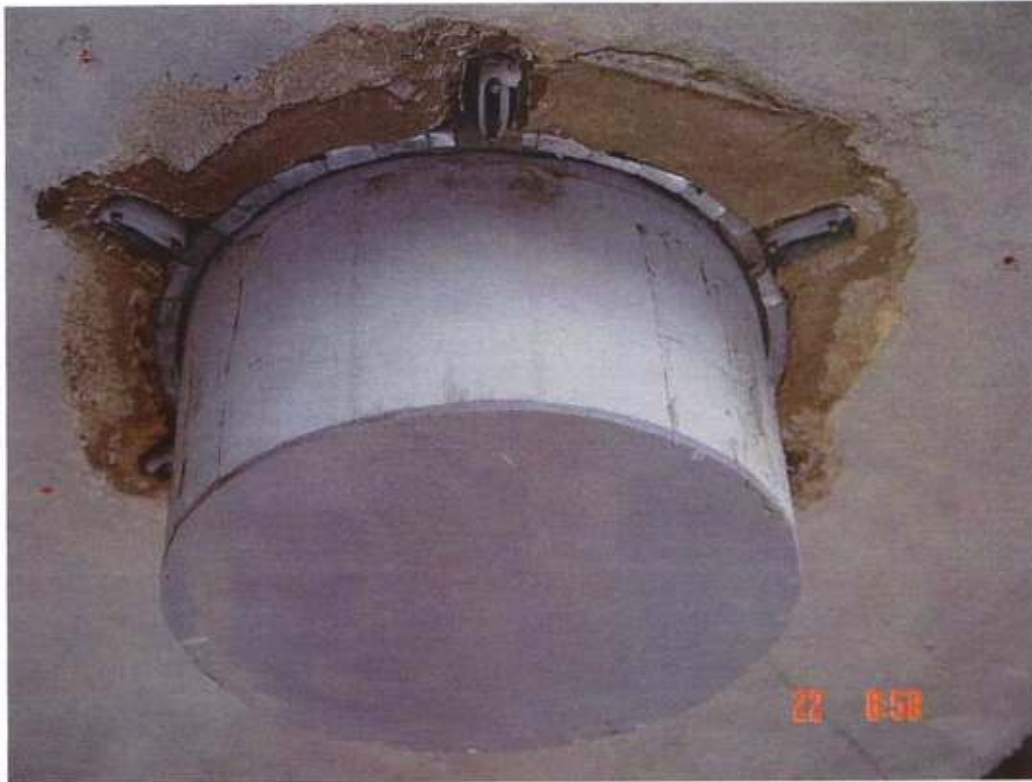
Photograph 1 - Specimen (exposed side) prior to testing.
